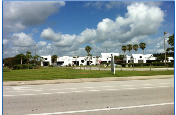
Grove Elementary School – immediately south of Site
